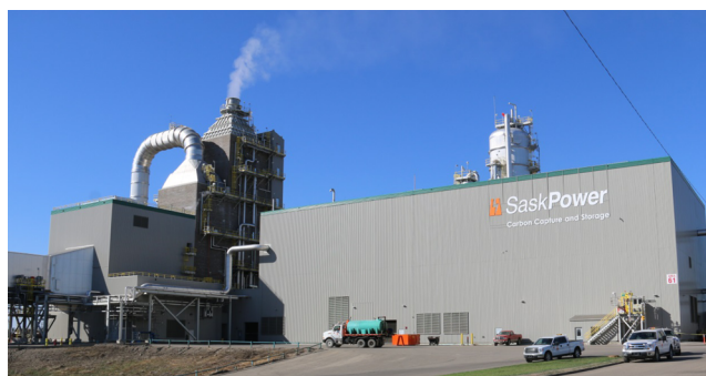
The first commercial scale carbon capture project captures CO 2 from a 55-year old coal-fired plant near Estevan, Saskatchewan, and stores it in nearby underground sites. Credit: SaskPower.
